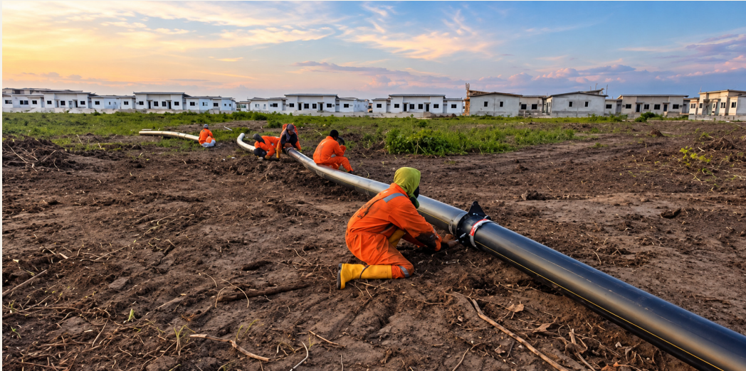
03 Crew positioning and connecting the pipeline across the site.
