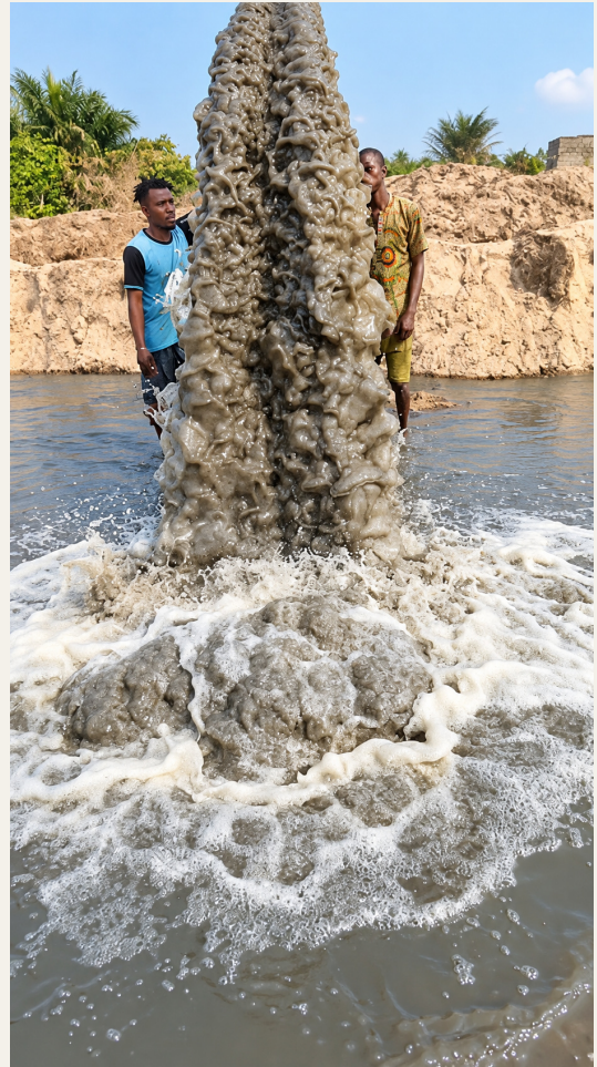
12 Discharge flow and receiving area at a sand-winning site.
