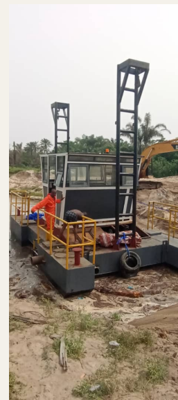
04 Compact pontoon and lifting frame positioned at the edge of a working site.
