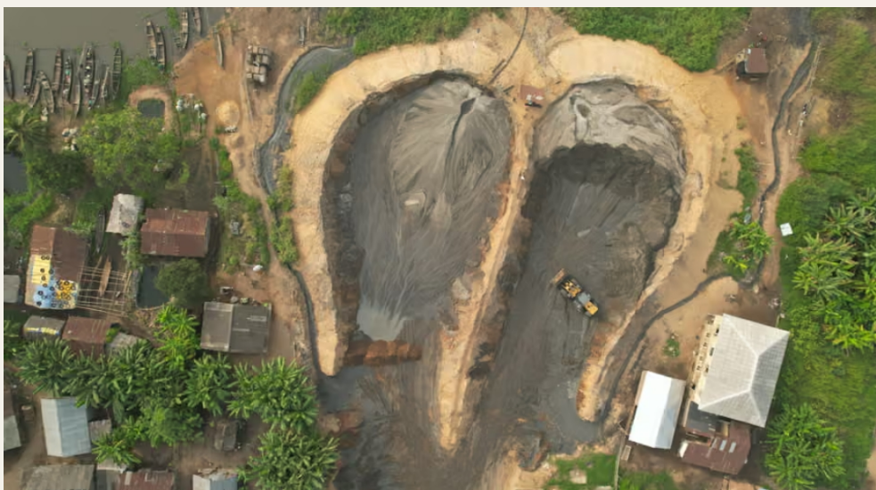
Aerial view of sand stockpiles and the surrounding working area.
