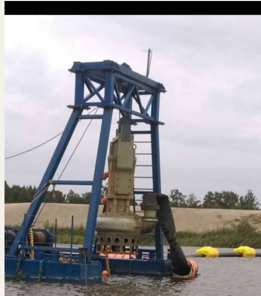
02 Suspended pump and lifting frame with a discharge hose leading away from the pontoon.
