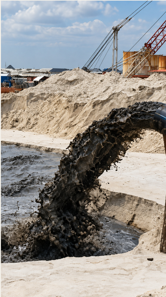
10 Hydraulic slurry discharge into a sand stockpile area.
