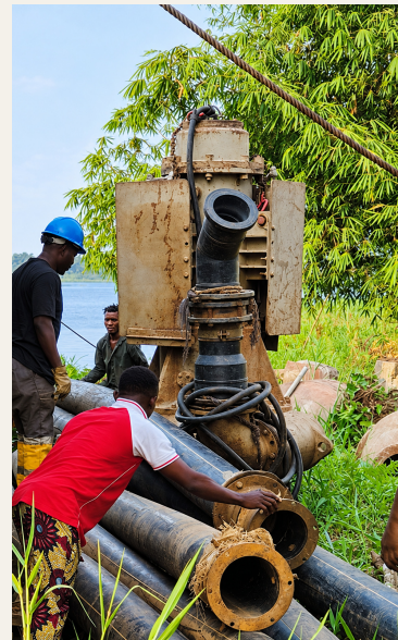
09 Crew preparing a pump and pipe connections before deployment.
